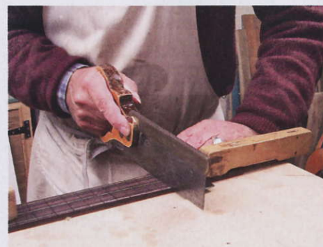
STEP 1. Cutting the fret slots
