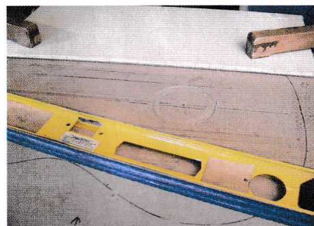
57 Pencil marks help to show when the butt join is perfect
